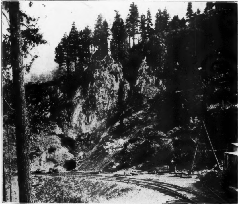
Showing the Trap Tunnel and Working Face of Quarry
